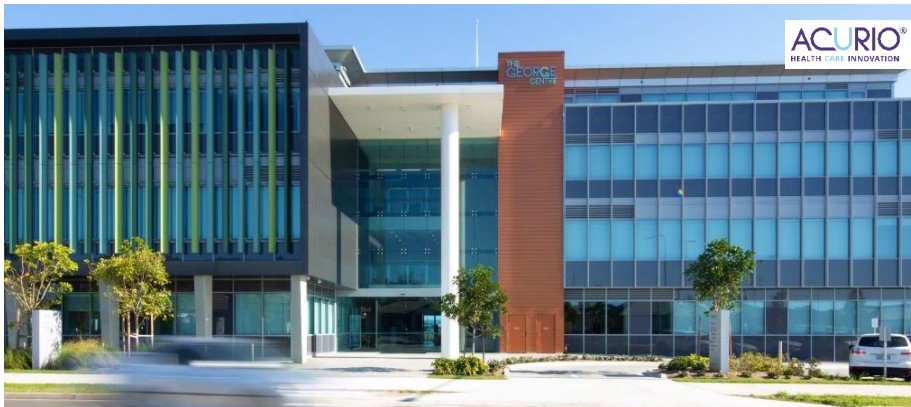
Knox Private Hospital (VIC) 3 – stage 1
